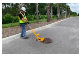
5.2.5 Step 5 Reposition pivot to the remoal position. Push forward to remove magnet.
